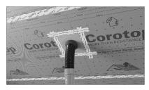
4. Seal all places where service lines pass through the vapour control layer (e.g. electrical cables, pipes, etc.) thoroughly with special adhesive or adhesive tape (e.g. Corotop FIX, Corotop BUTYL).
