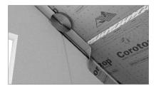
3. The places where vapour control layer connects to the wall should be sealed with special adhesive or butyl tape (e.g. Corotop BUTYL). It is recommended to use an additional hold down strip and to leave about 2 cm of excess foil (folds).
